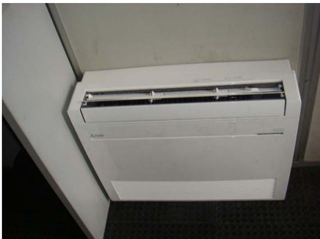
FIG. 17 – UNITÀ INTERNA SISTEMA DI EMERGENZA
